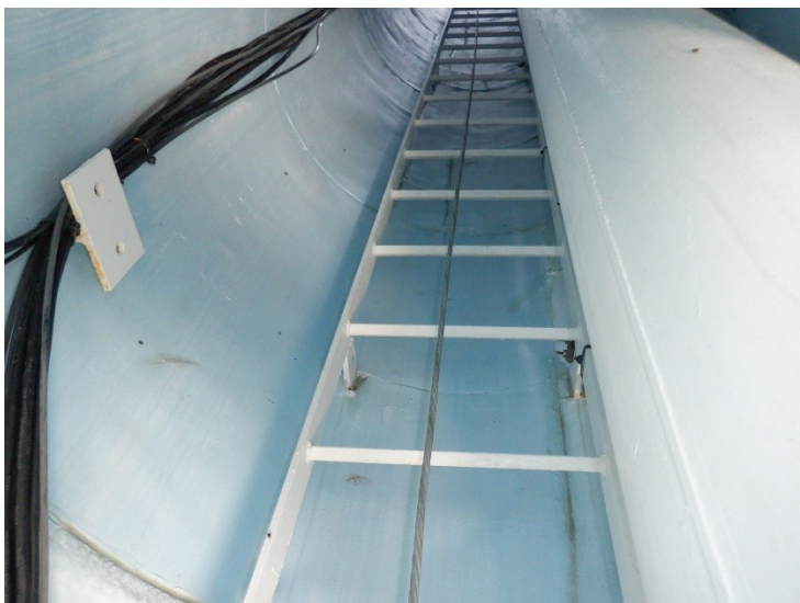
66) The access tube ladder is in good condition. The ladder is equipped with a fall prevention device.
