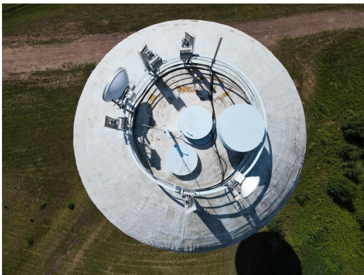
30) The roof handrail is being used for antenna mounting.
