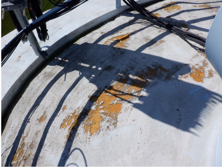
25) The insulation on the roof has deteriorated.
