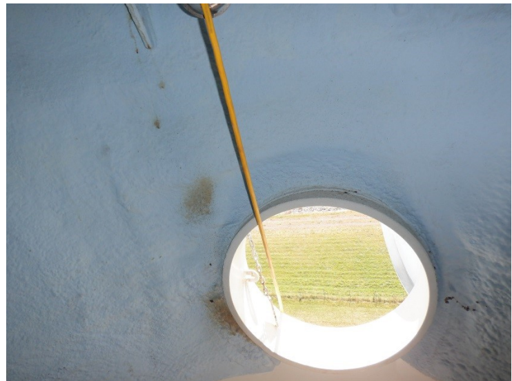
59) There is no handhold above the painter's hatch at the top of the riser.
