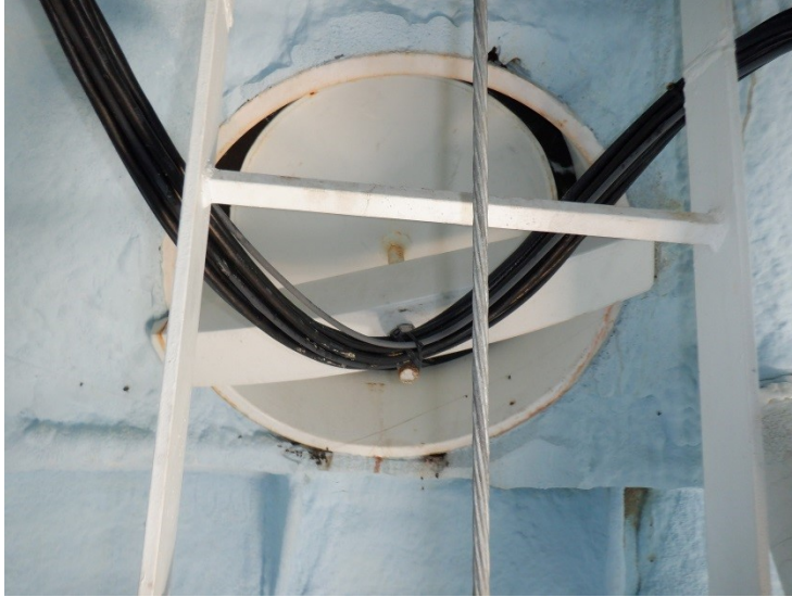
61) The wet interior manway in the transition cone is in good condition.
