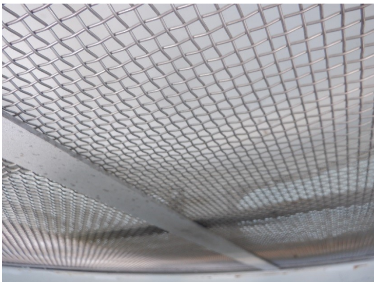
39) The interior roof vent screen is in good condition but oversized.
