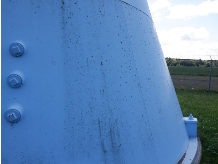
10) There are a few minor coating failures on the basebell.
