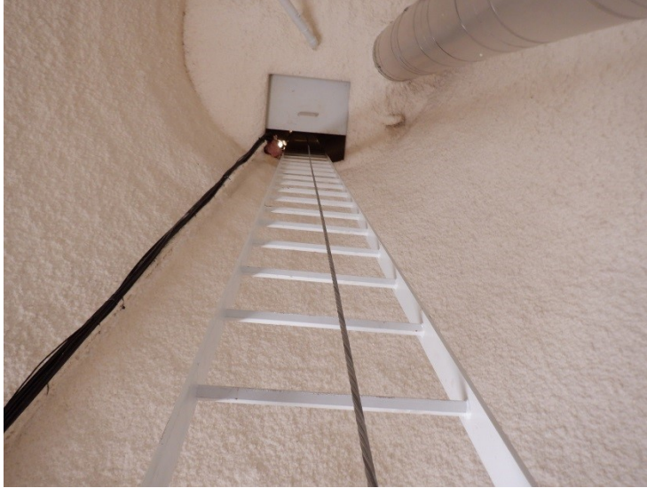
46) The basebell ladder is in good condition. The ladder is equipped with a fall prevention device.
