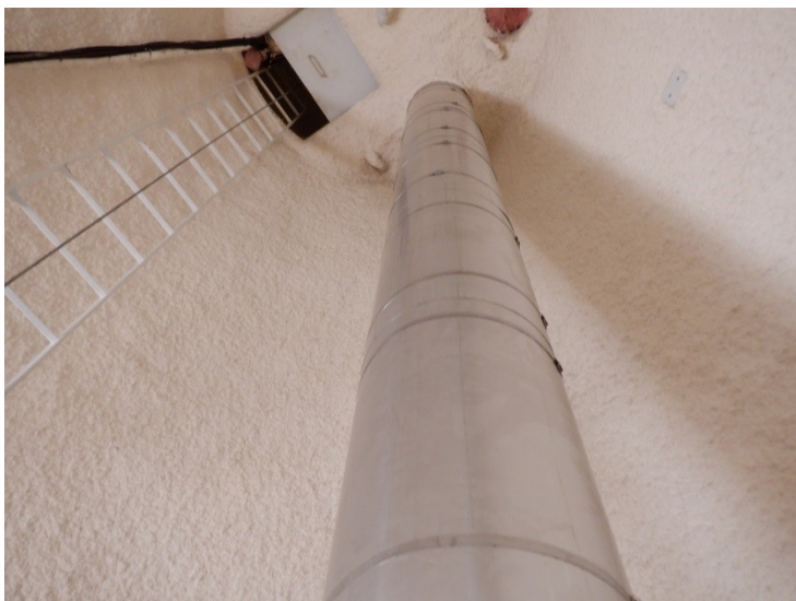
45) The fill/draw pipe insulation and aluminum cover are in good condition.
