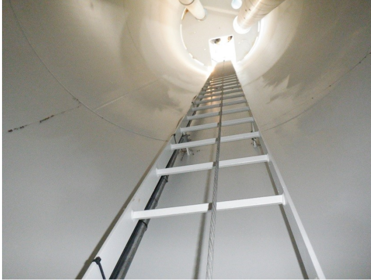
55) The riser ladder is in good condition. The ladder is equipped with a fall prevention device.
