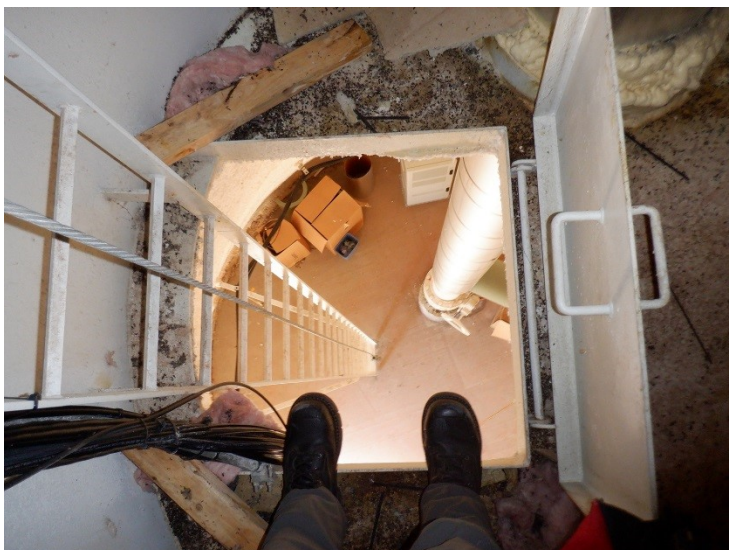
48) The ladder opening in the condensate platform is equipped with a hinged cover.
