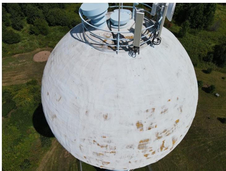
27) The coating on the roof insulation is in fair condition with areas of erosion.
