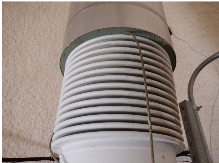
44) The bellows expansion joint on the fill/draw pipe in the basebell appears to be in good condition.
