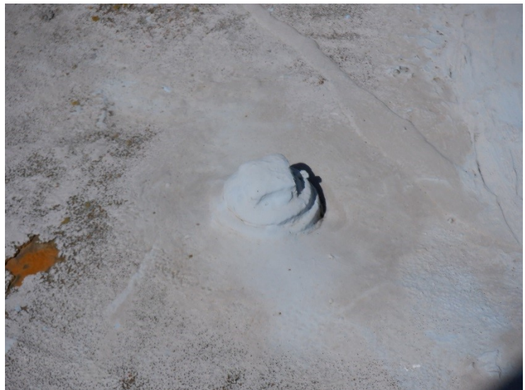
35) The roof rigging couplings are properly capped.
