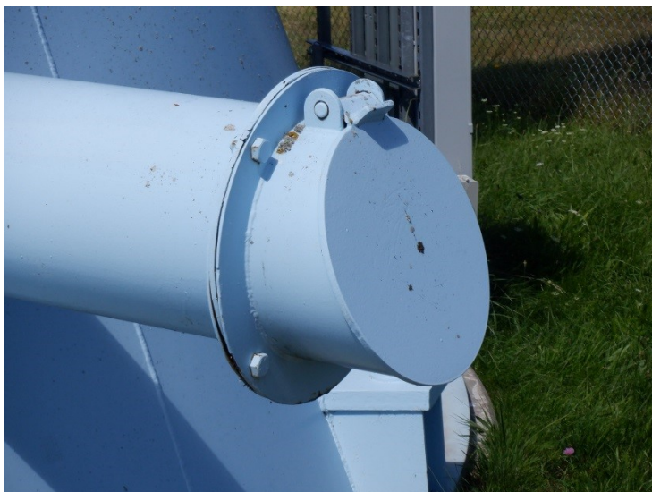
6) The solid flap gate at the overflow pipe discharge operated properly.
