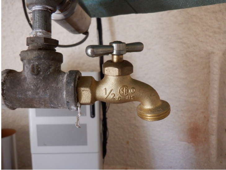
43) The sample tap on the fill/draw pipe in the basebell has a threaded end.
