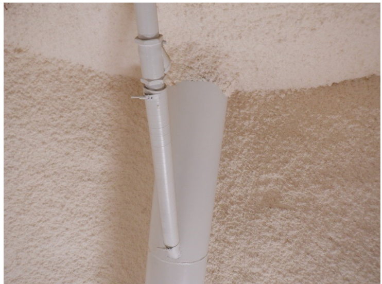
47) The condensate platform drain with a check valve is in good condition.
