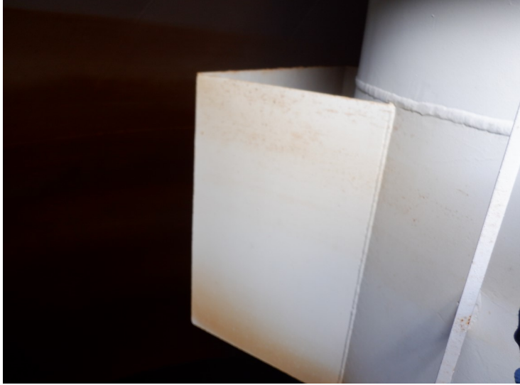
79) The overflow pipe weir box at the top of the access tube is in good condition.
