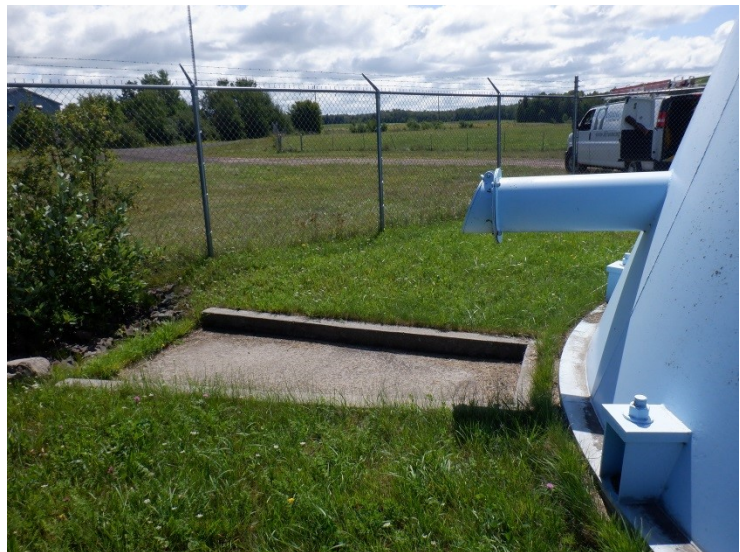
5) The overflow pipe discharges to a concrete splash pad and riprap.
