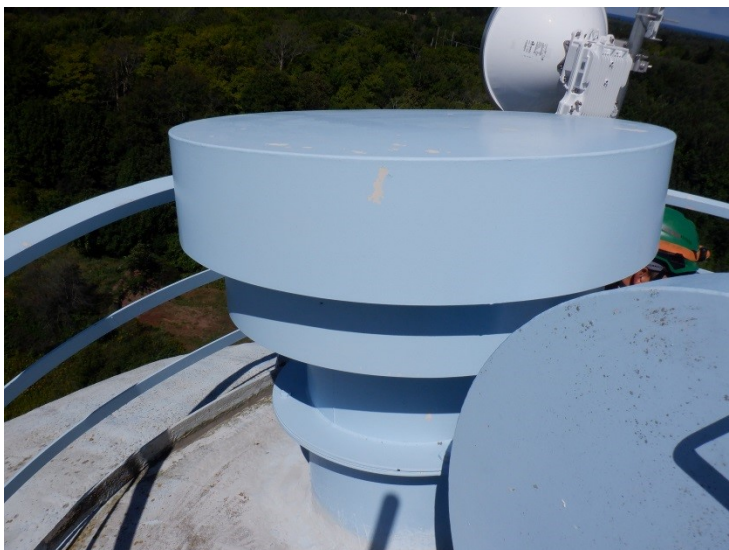
36) The pressure vacuum roof vent is in good condition.
