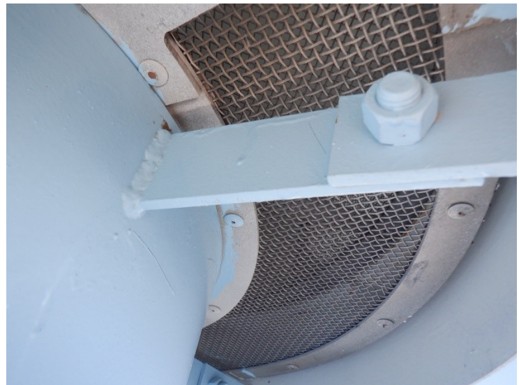
38) The screened roof vent pressure plate was found to be properly aligned.
