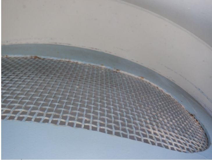
37) The external roof vent screens are in intact.
