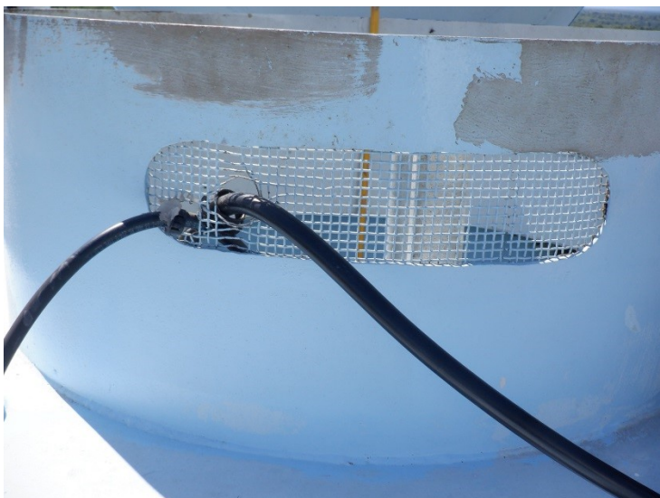
33) Antenna cables are routed through the screens on the access tube roof hatch neck. The screen are oversized.
