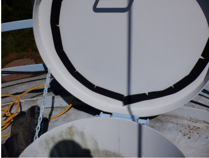
34) There is a gasket on the wet interior roof hatch.
