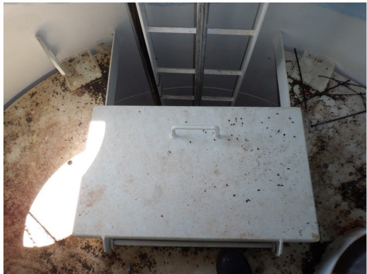
56) The ladder opening in the top platform is equipped with a hinged cover.
