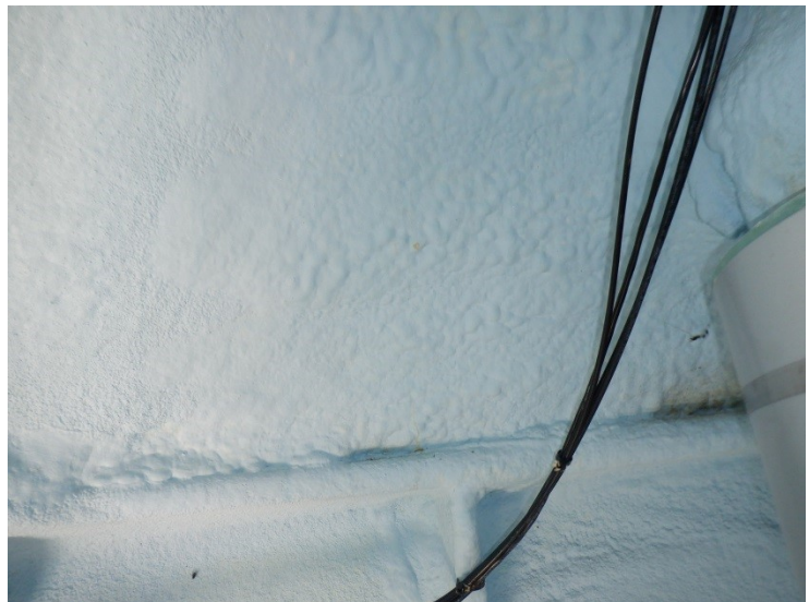
62) The transition cone coating is covered with spray foam insulation and not visible for inspection. The insulation is in good condition.
